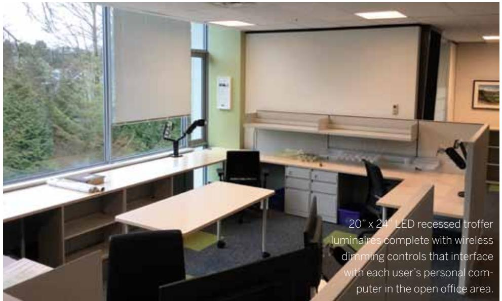
interfaced with each user's personal computer in the open office areas. Set at 50 per cent dimmed, these luminaires achieve a lighting power density of 0.18 watts per square foot, exceeding ASHRAE 90.1/2010 LPD requirements by 80 per cent, while still meeting industry target illumination levels.
